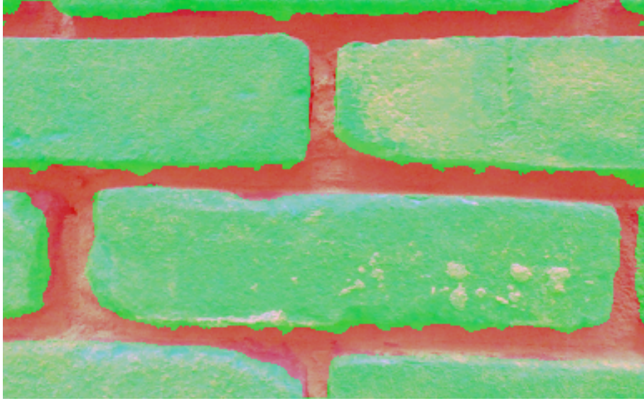
Figure 4.7: Labeled frame (Joint: Red, Brick: Green)
